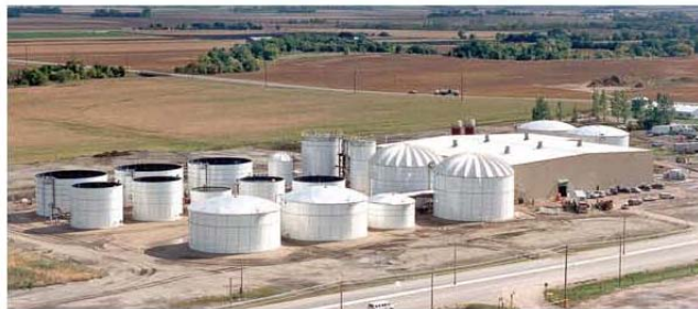
Anaerobic Digester Facility, Minnesota
